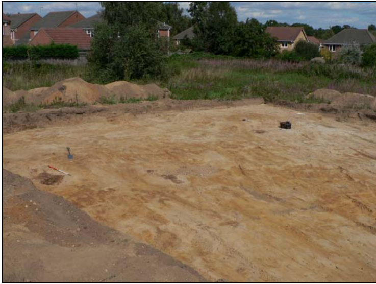
Excavation area from southwest
