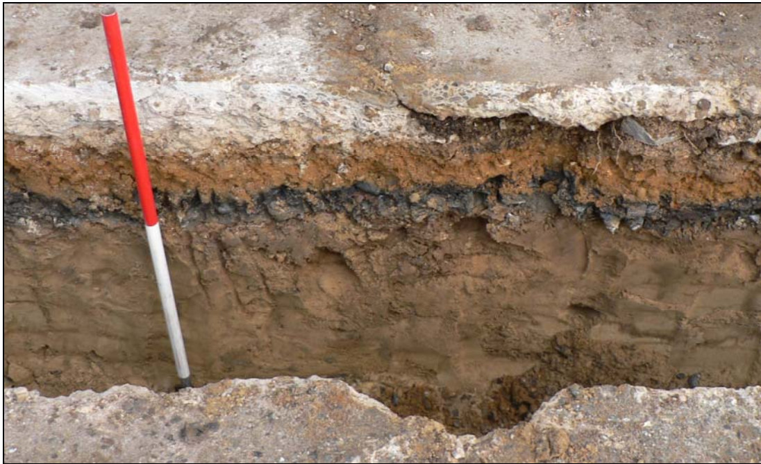
Image 2- area 1, former cattle shelter, concrete surface over hoggin & cobbled surface
