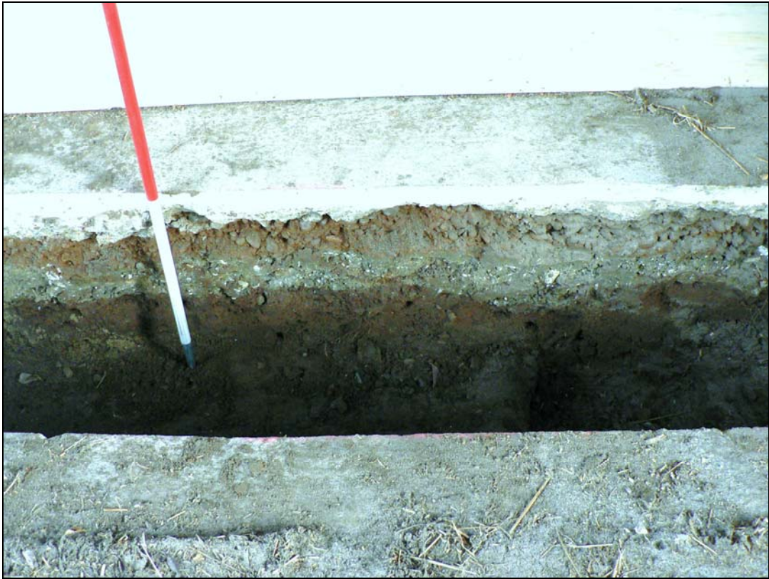
Image 3- clay floor below concrete surface (taken under indoor lighting)
