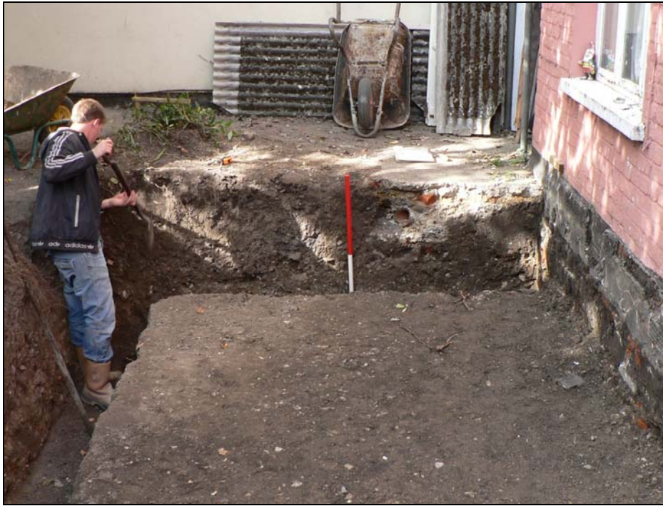
Front extension footings under excavation
