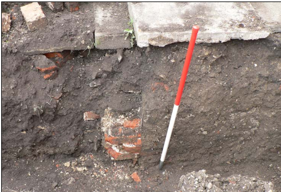
Eastern footing trench to rear extension with wall 0002 & 0001 to left & 0003 to right
