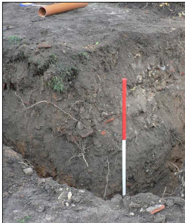
Rear extension footing trench from north-east
