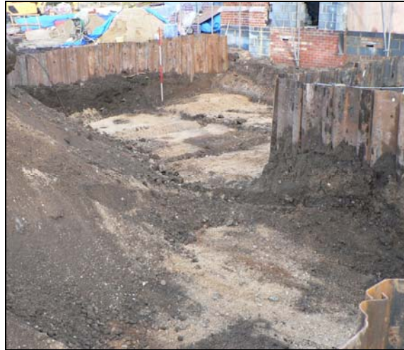
Cellar excavation from south-west
