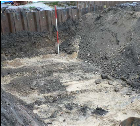
Cellar excavation from north-east
