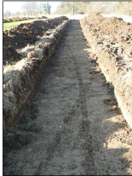
Trench 2 from west with field drains
