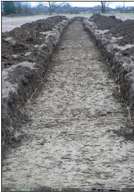
Trench 5 from west
