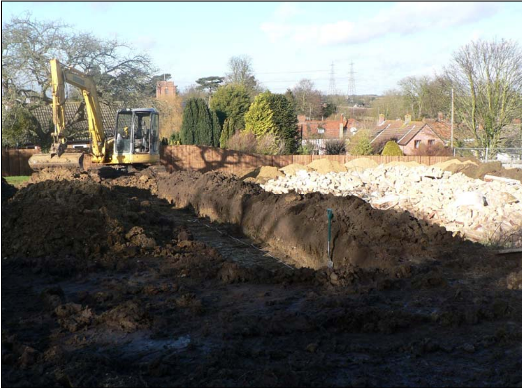
General view from south with trench 3 in foreground & church in background
