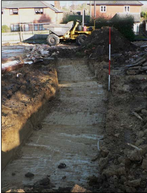
Trench 2 from west
