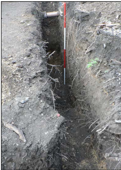
Northern trench & pit 0002 from west
