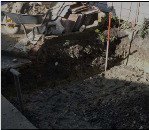
Western trench from south-east
