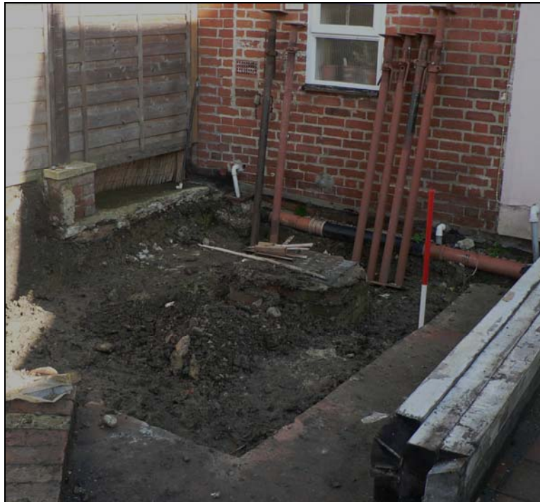
General view from south-west
