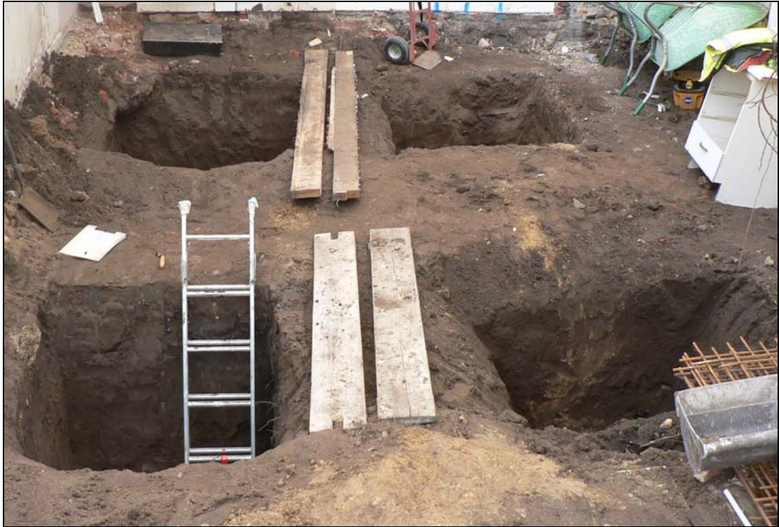
Pad foundations at the rear of the house from the north-west
