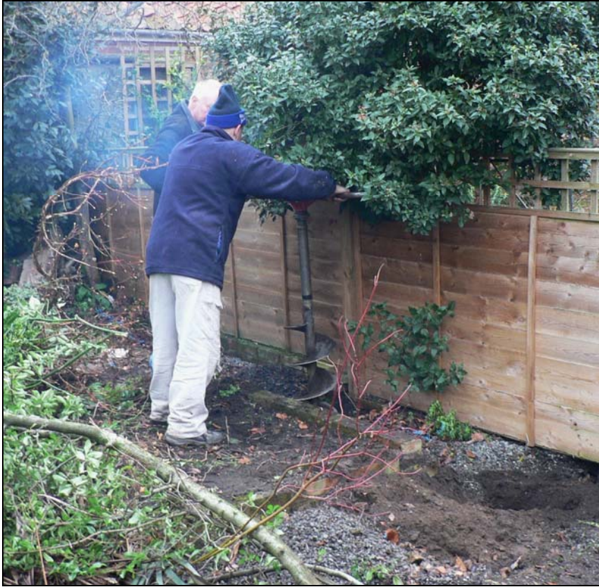
Boring of foundations for the garden room
