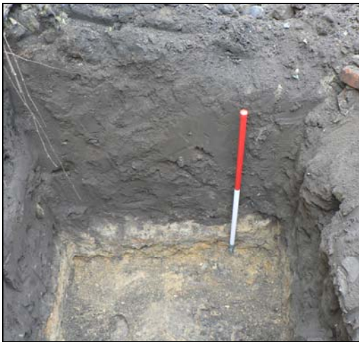
North-western pad foundations
