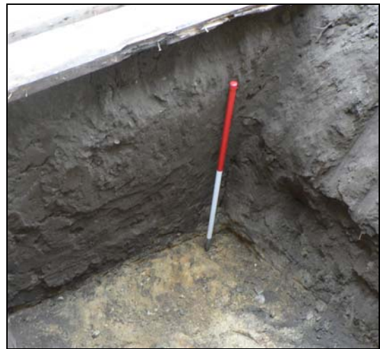
South-eastern pad foundation
