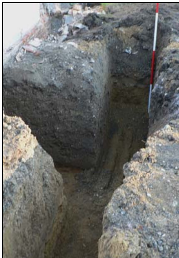
Eastern footing trench from north
