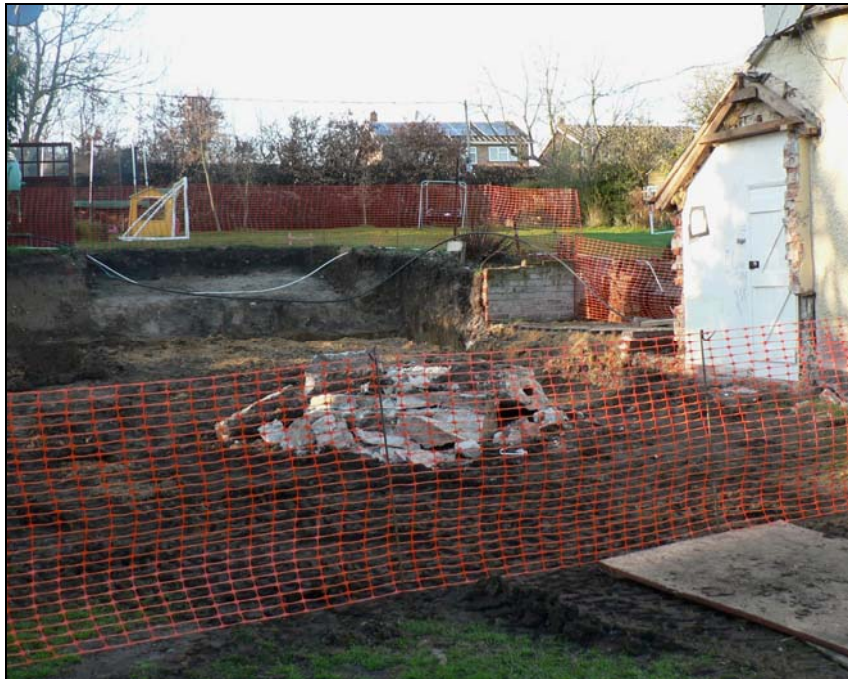
General view from south-west showing terraced footprint area
