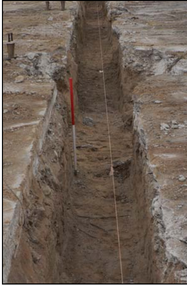
Southern foundation trench to new car showroom
