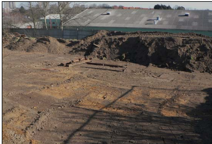
Area stripped for car in north-eastern quarter of the site
