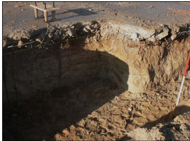
Eastern foundation trench to new car showroom
