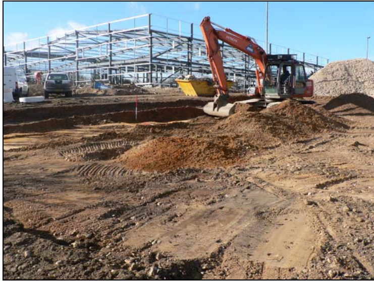
General view of site from south-east
