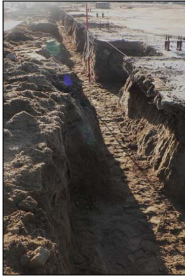
Western foundation trench to new car showroom
