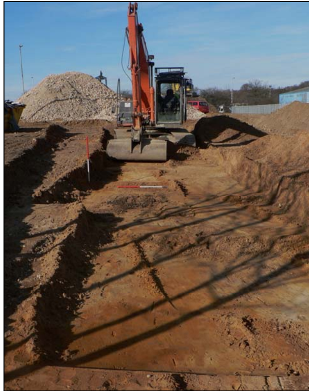
Soil stripping for storm water tank area
