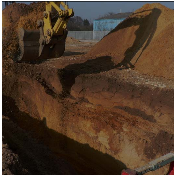
Pipe trench crossing line of cropmark anomaly from south-west
