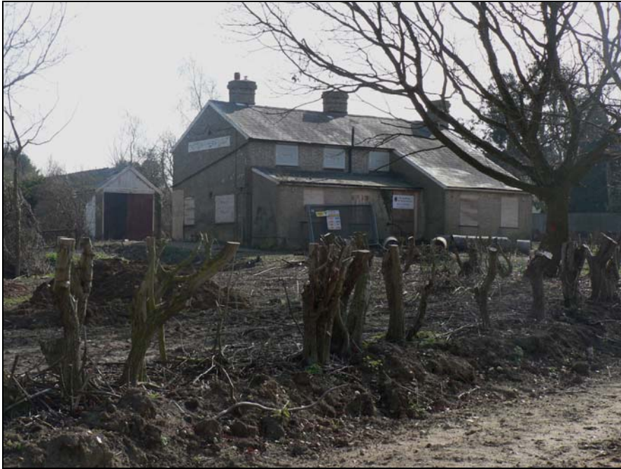
General view of PH buildings from north-west
