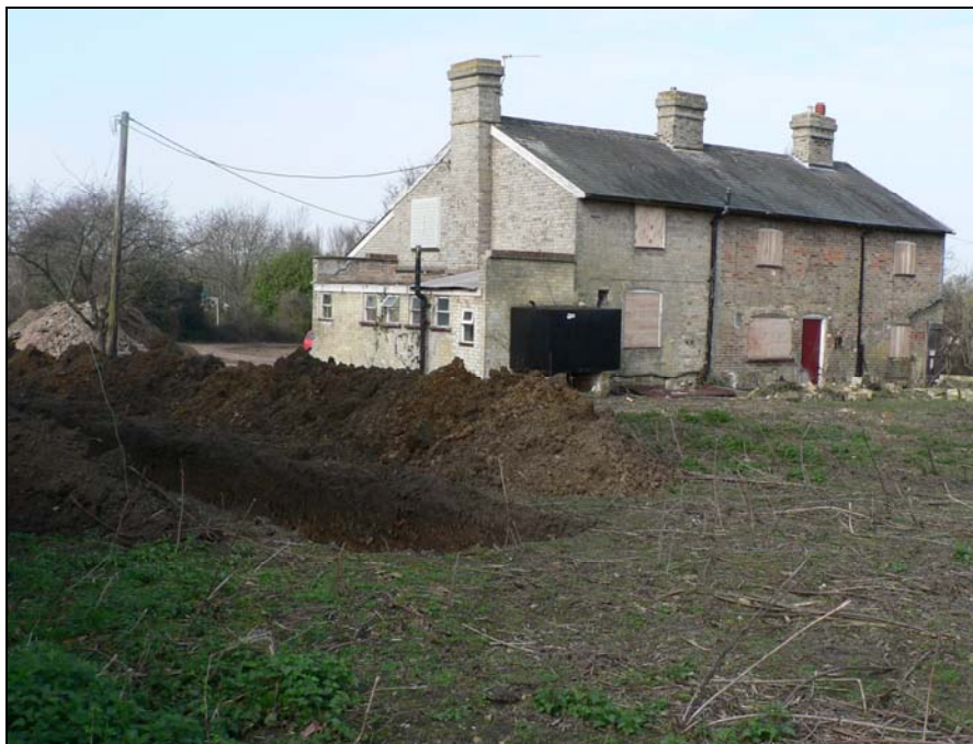
General view of PH buildings from south-west
