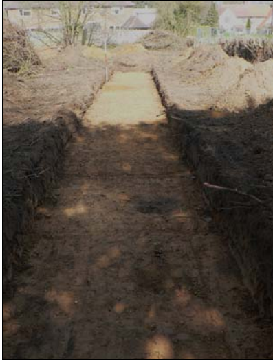
Trench 1 from south
