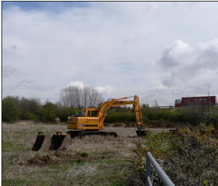
General view across site from south-west corner
