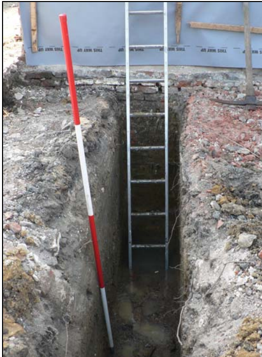
Footing trench showing house foundations
