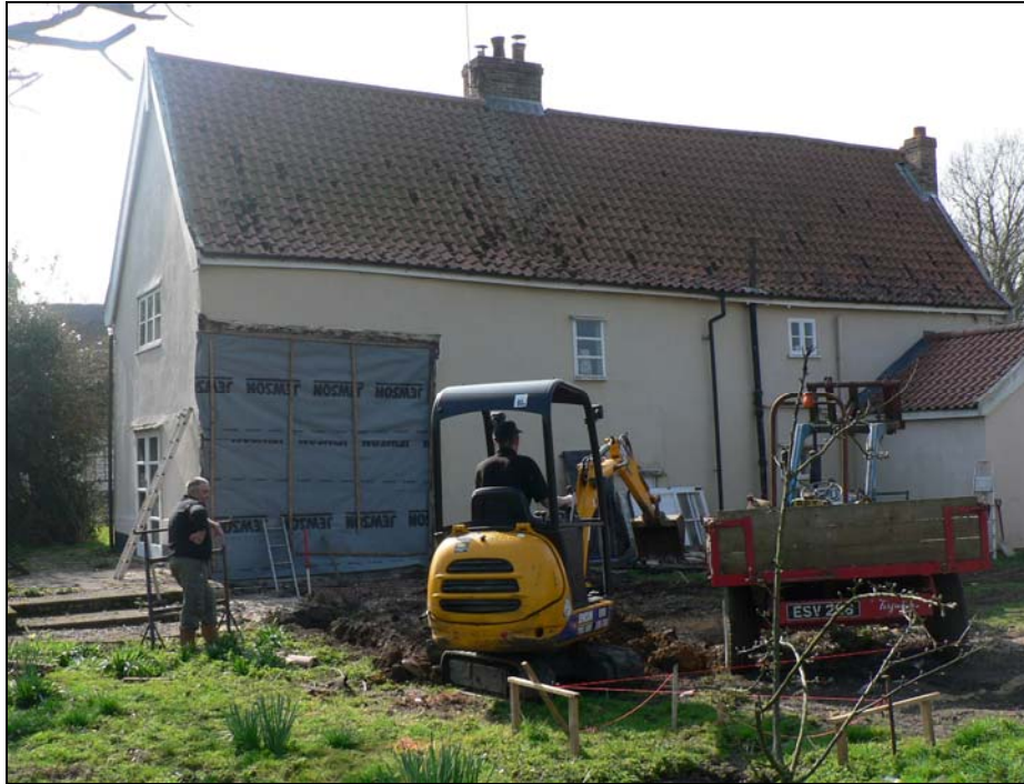
The rear of Lavender Cottage from north-east
