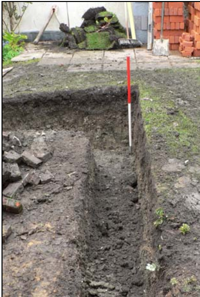
South-eastern corner of footings
