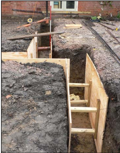
Eastern footing trench from south
