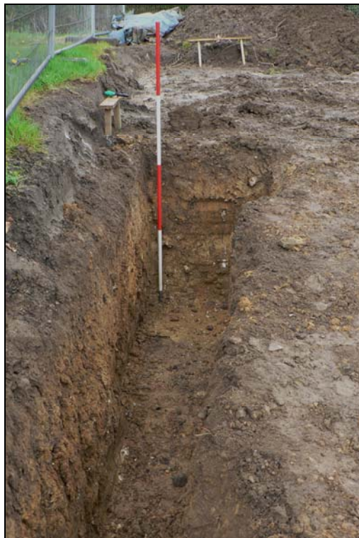
Eastern footing trench from north
