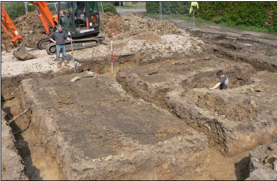
Footings from south-west
