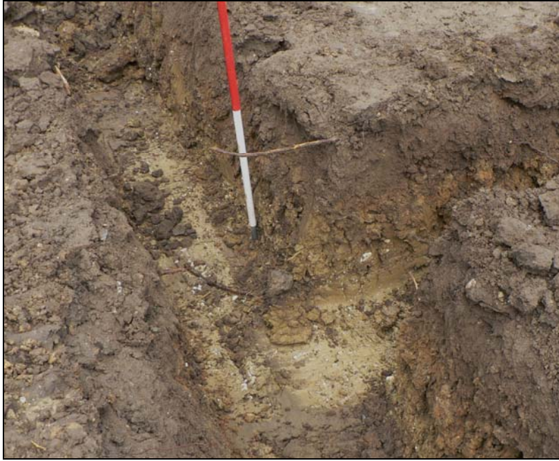
Central footing trenches
