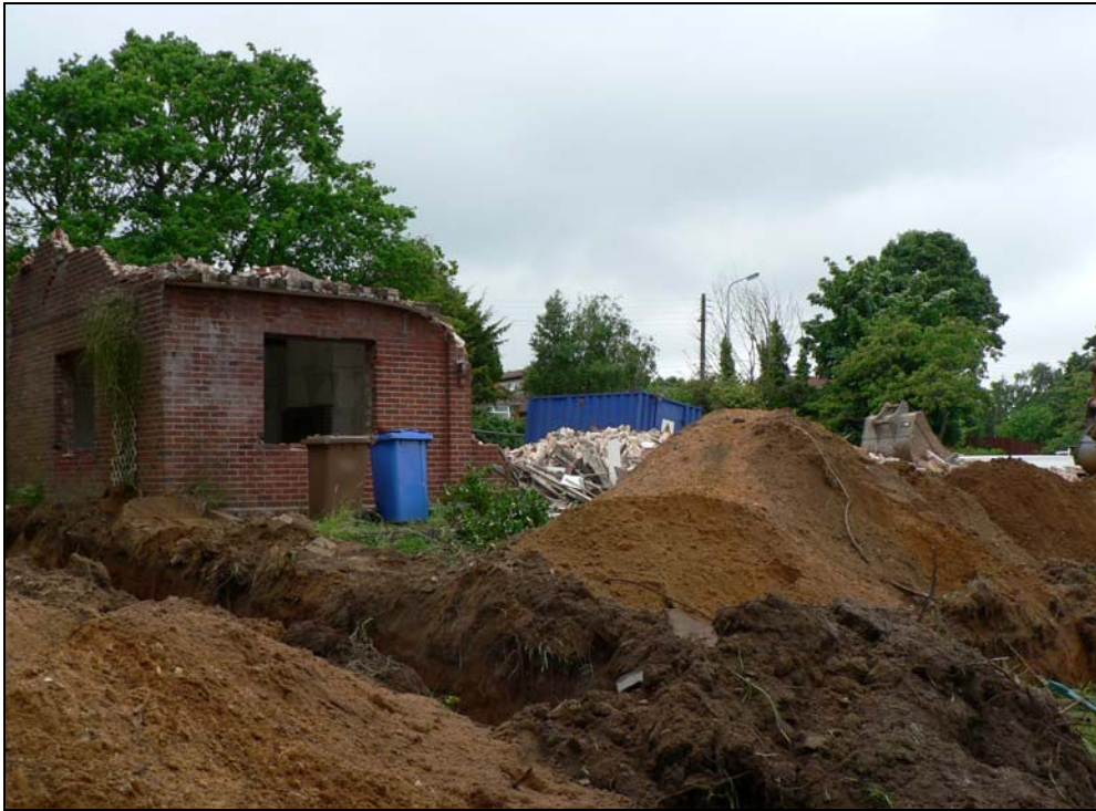
General view from south-east
