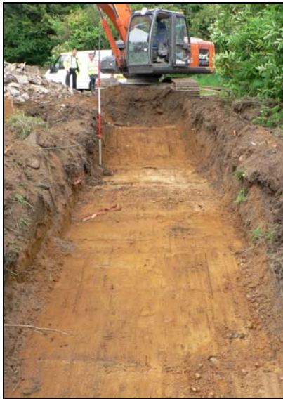
Trench 1 from east
