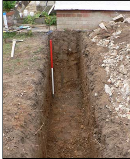
Western extension footing trench
