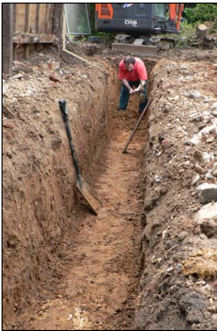
Eastern extension footing trench from north
