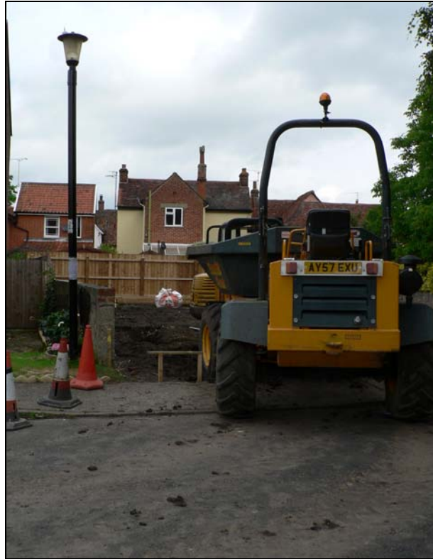
General view from south (64 Angel Street in background)
