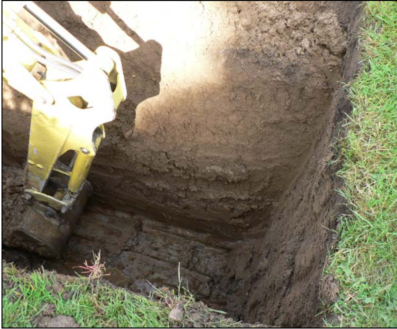
Septic tank pit under excavation
