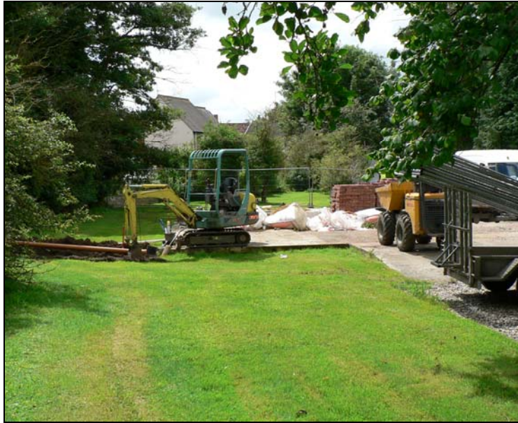
General view from north
