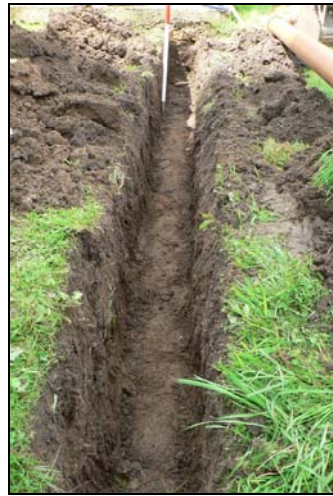
Northern pipe trench from east
