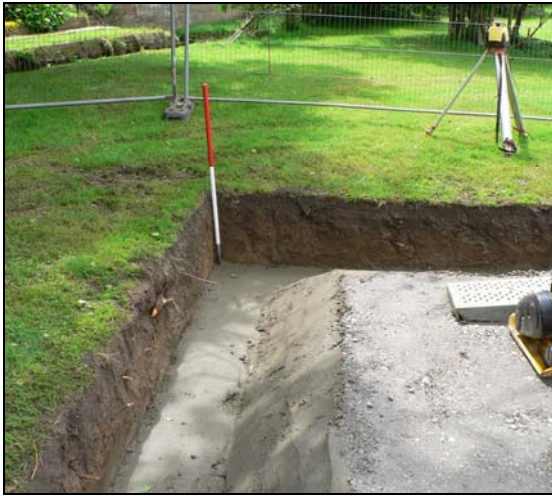
Southern section of slab foundation area
