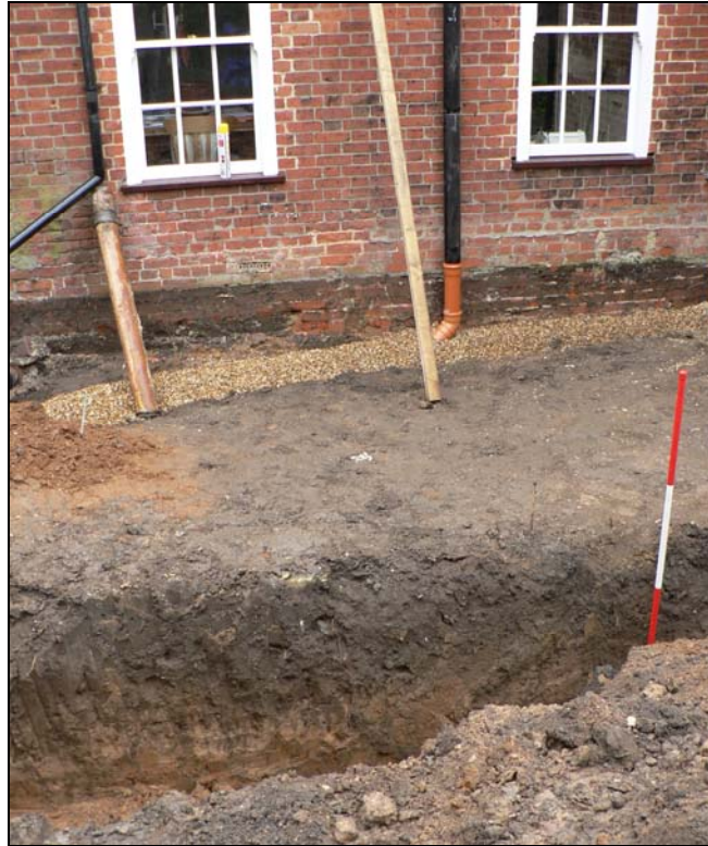
Extension area from west with house in background
