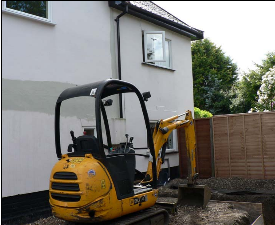
Site from north-east
