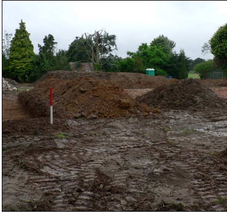
General view from northeast- green/golf course in background
