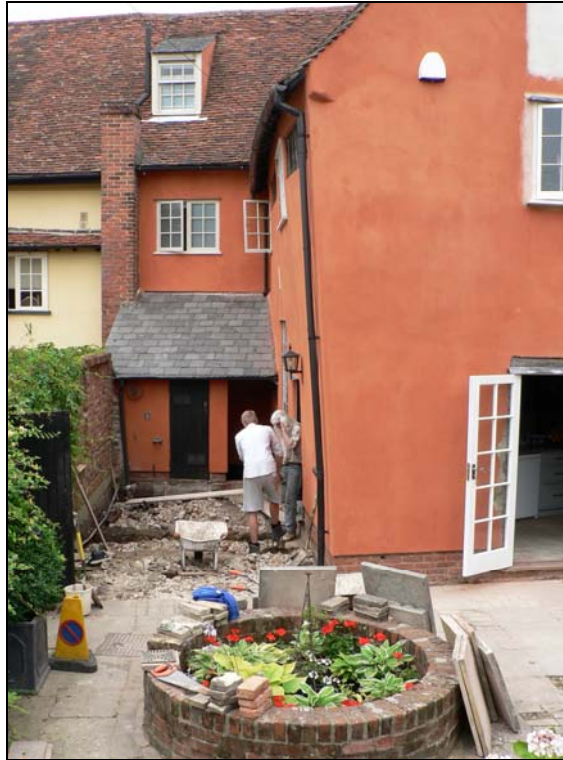
Extension area from back garden to east
