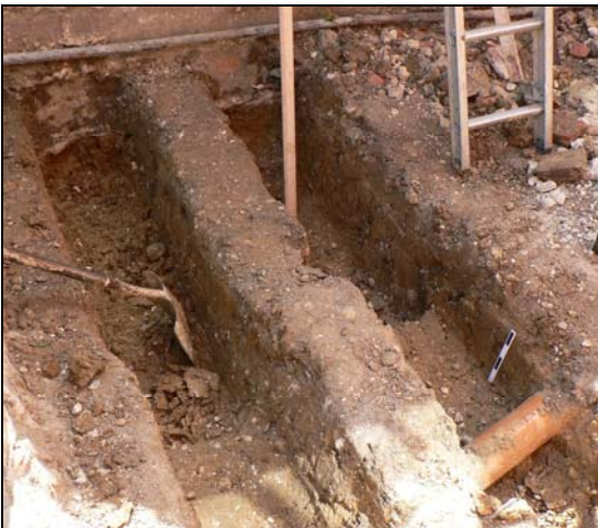
Eastern pair of foundation trenches
