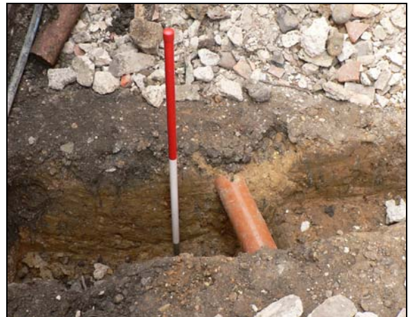
West central foundation trench
