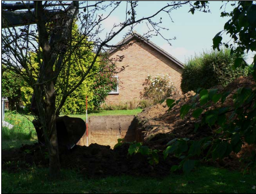
Site from south
