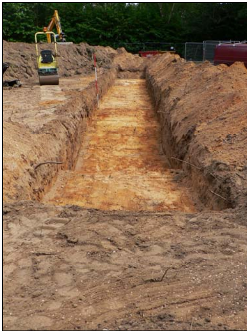
Trench 4 from west
