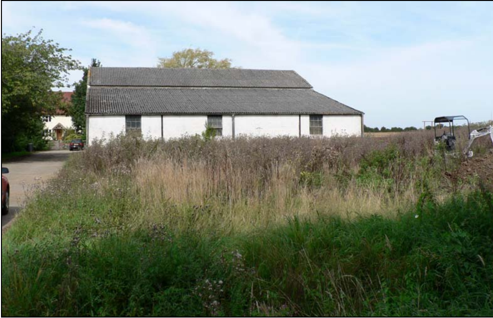
General view of site from south, Church Farm House left background
