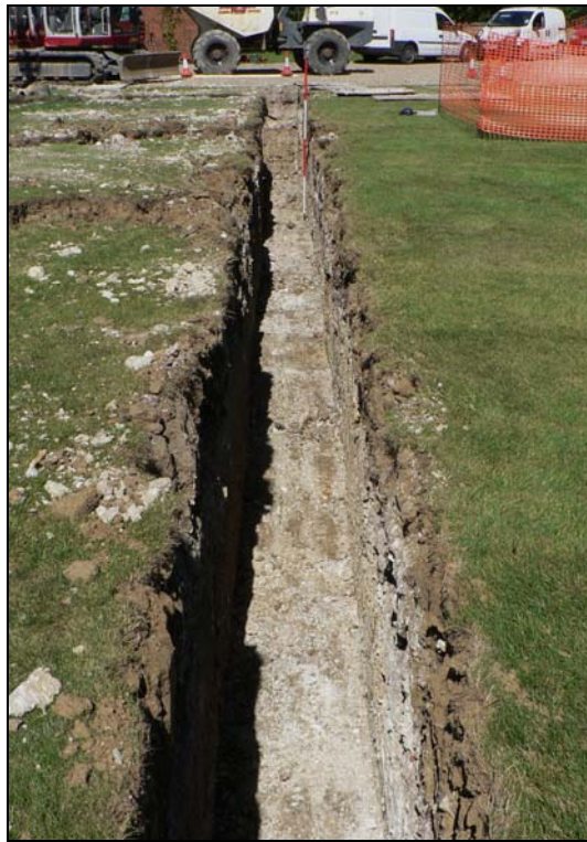
Eastern footing trench from south
