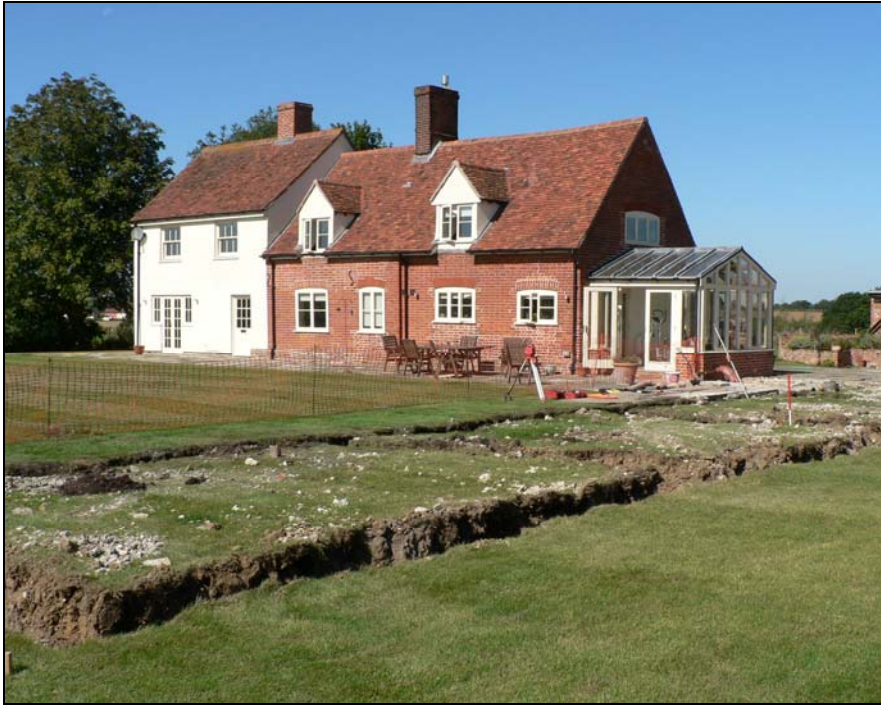
General view from south-east
