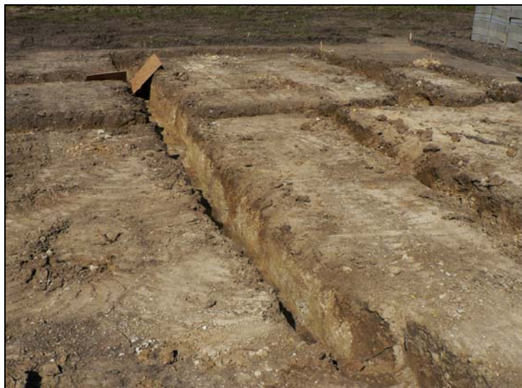
Excavated house foundations from east
