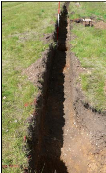
Monitoring- wall trench from east
