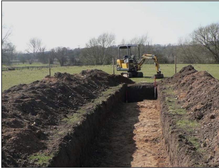
Evaluation trench from east
