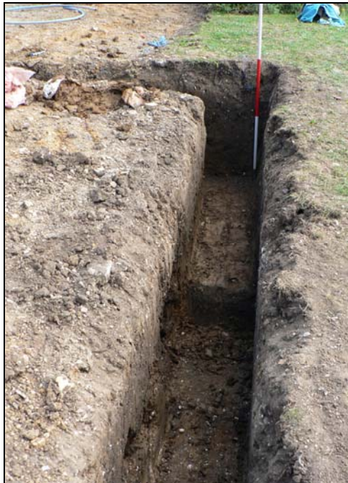
Southern foundation trench from east (modern soakaway feature in foreground)
