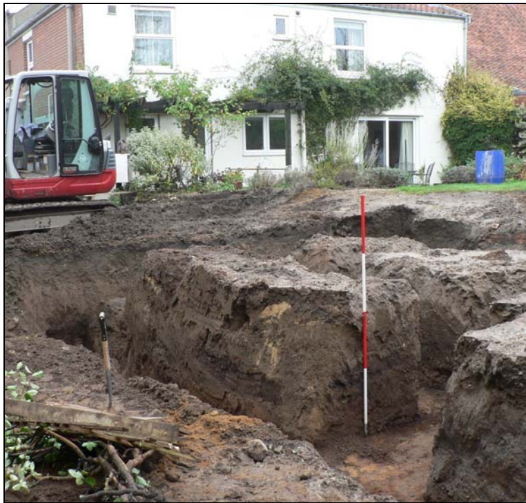
General view from north-west across footings, Post Office Cottage in background
