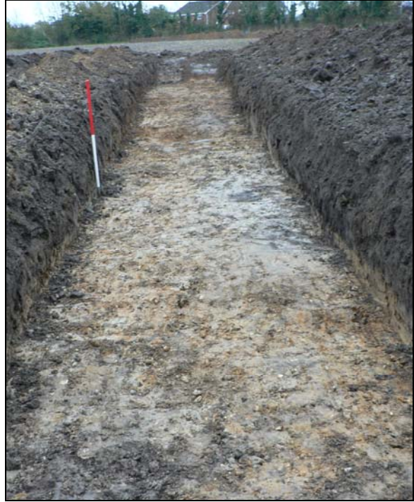
Trench 2 from west
