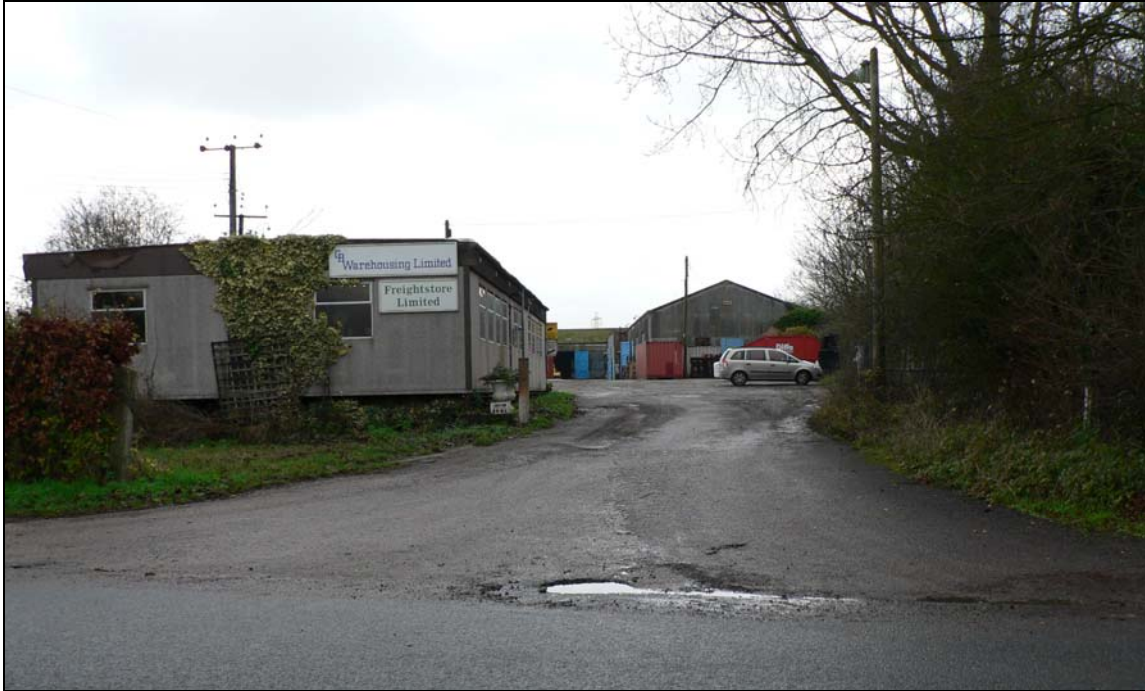
Northern part of site from east
