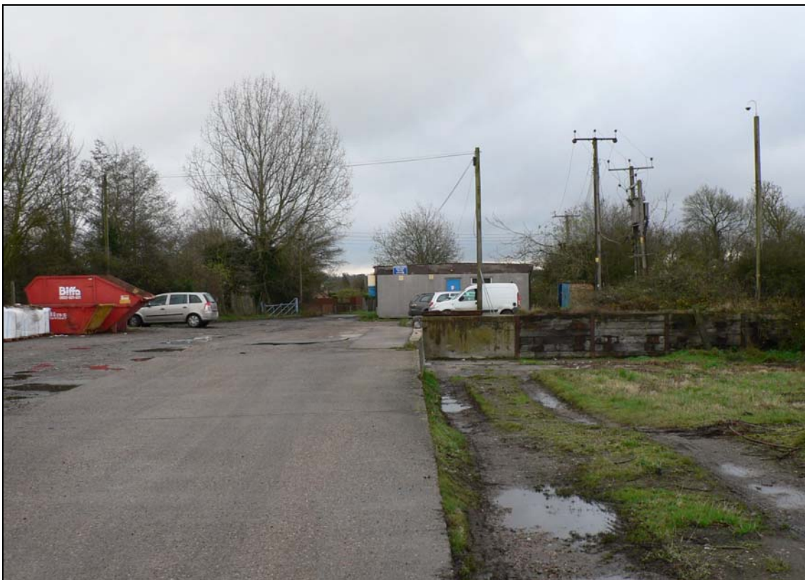
Northern central part of site, possible remnant of station platform centre foreground, ground truncation to right in area of former track
