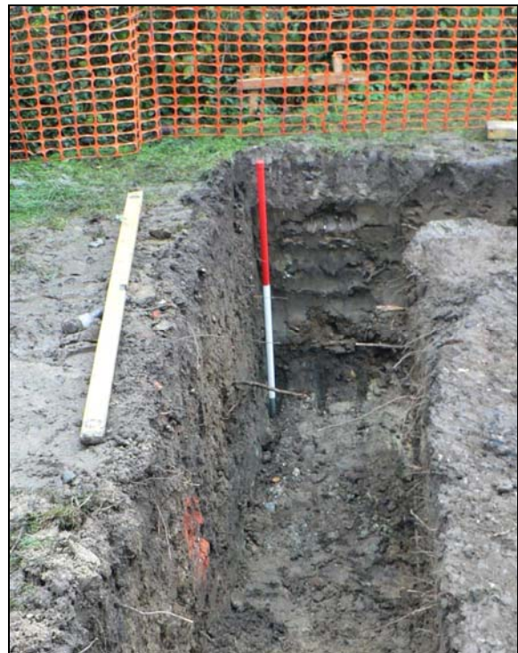
South-east corner of foundations
