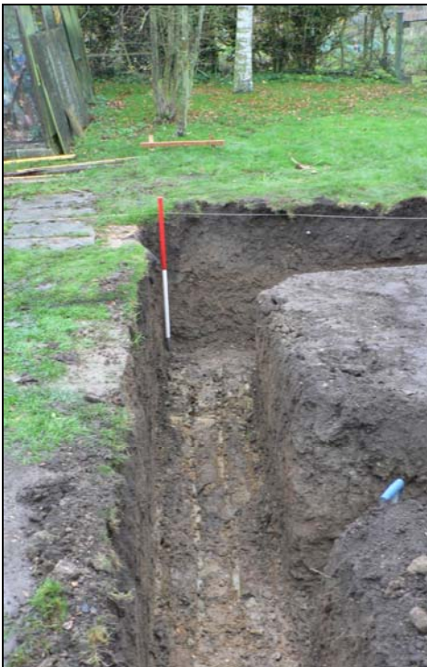
North-east corner of foundations
