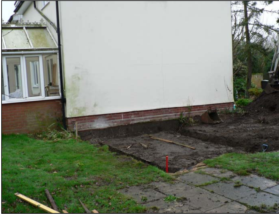
Site from north-east
