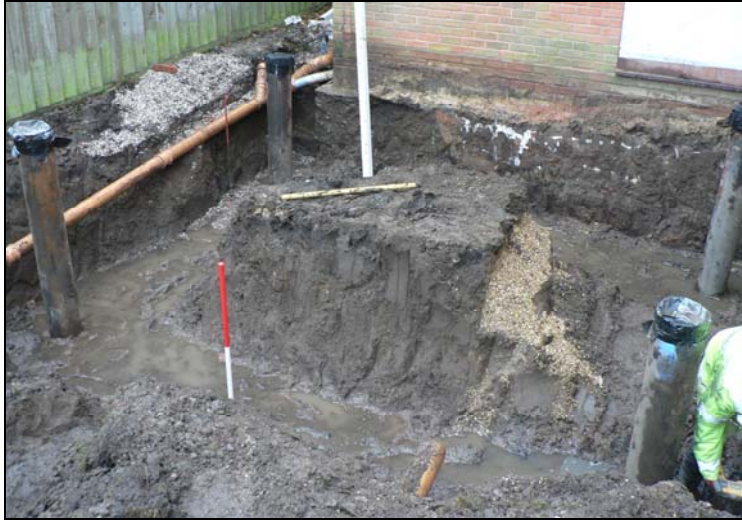
Fully excavated ground beam trenches from north
