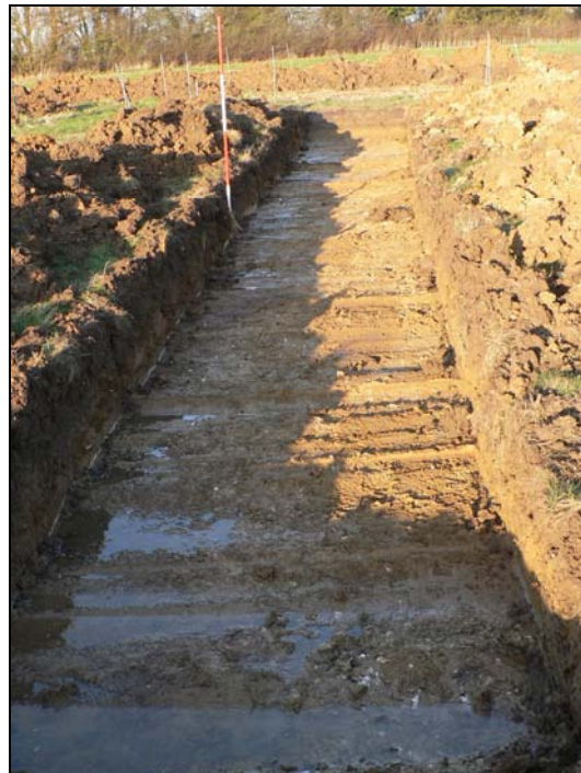
Trench 2 from south
