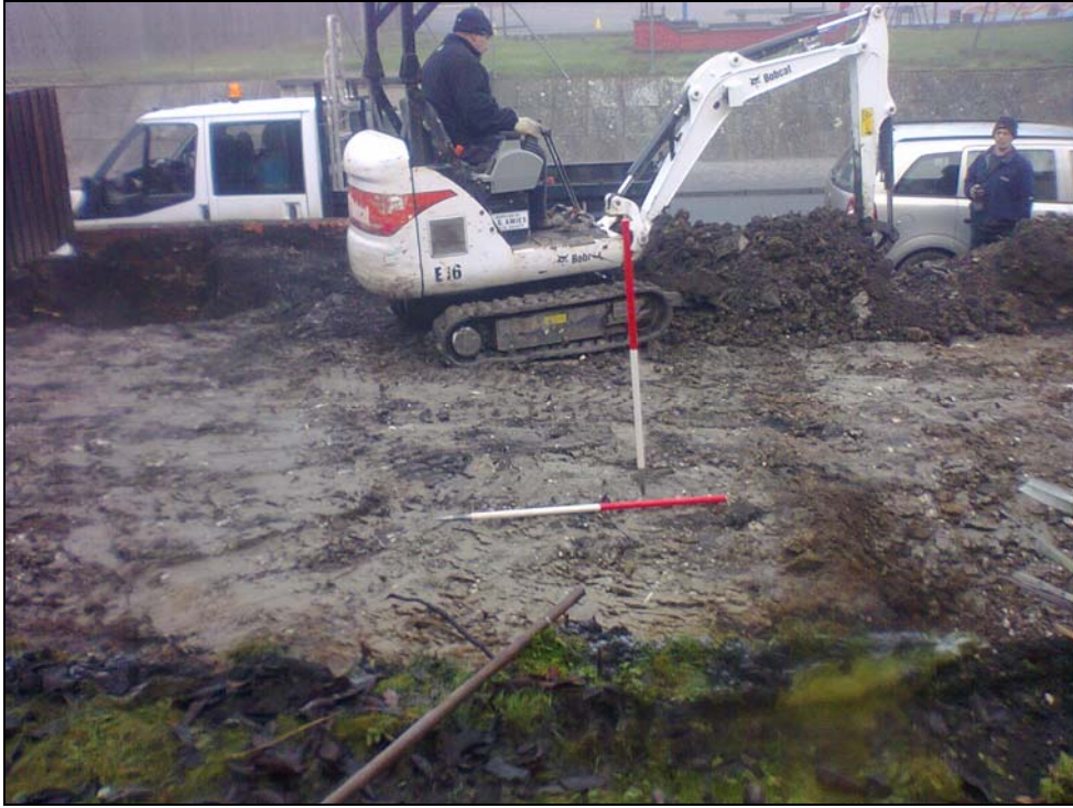
Stripped area from south
