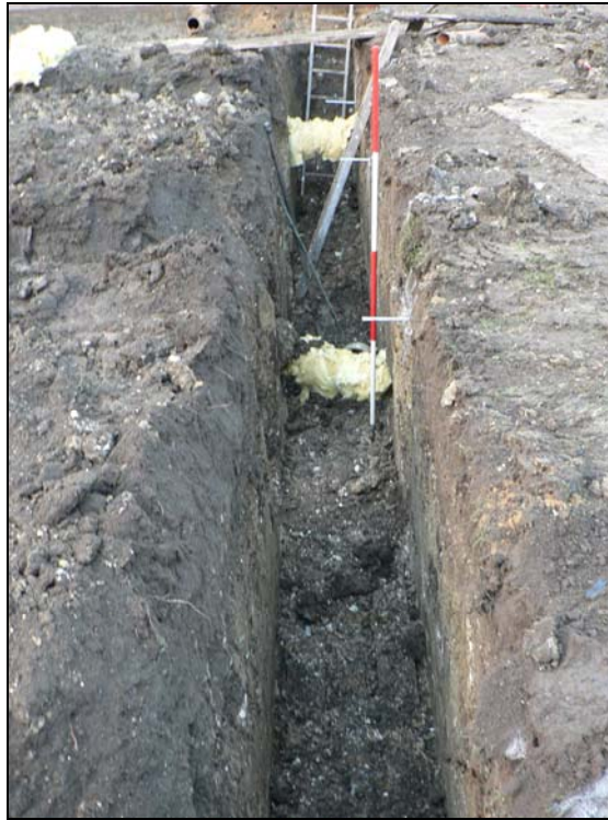
Eastern foundation trench from south
