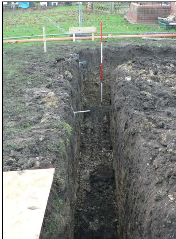
Southern foundation trench from east
