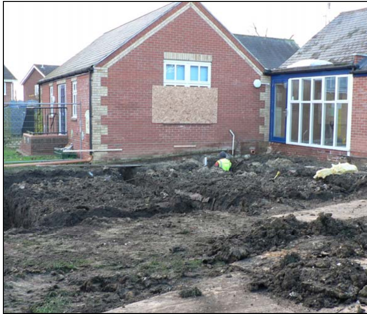
Area of new extension from south-east
