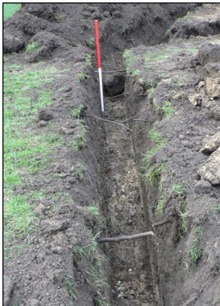
Drainage trench on western side of extension
