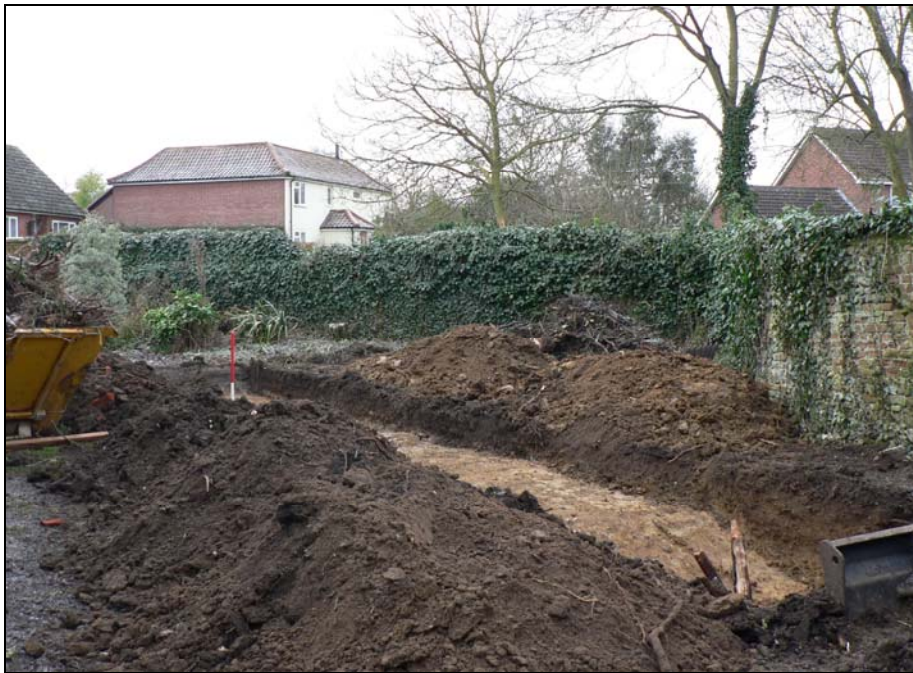
General view from north-east with flint wall in background
