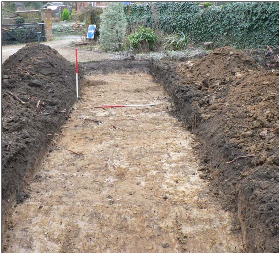
Trench from north
