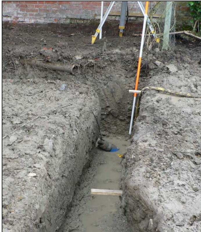
Deposit profile for conservatory footings
