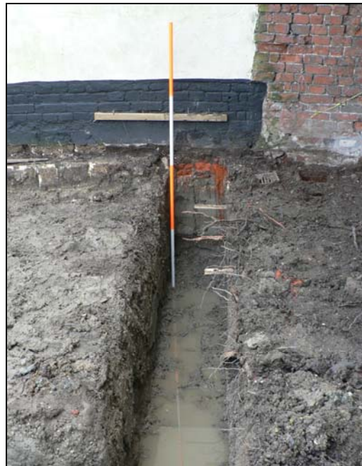
Western footing from north
