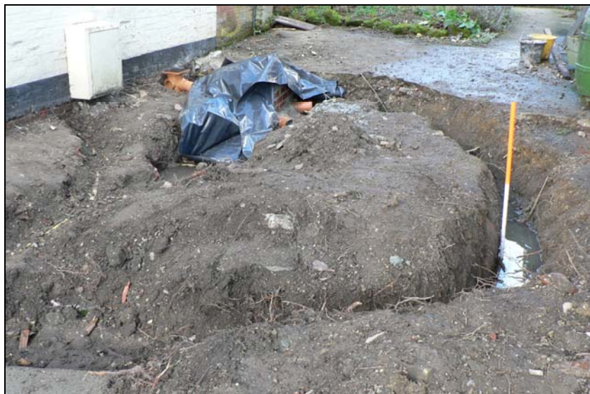
Entrance enclosure pipe diversion trench from south
