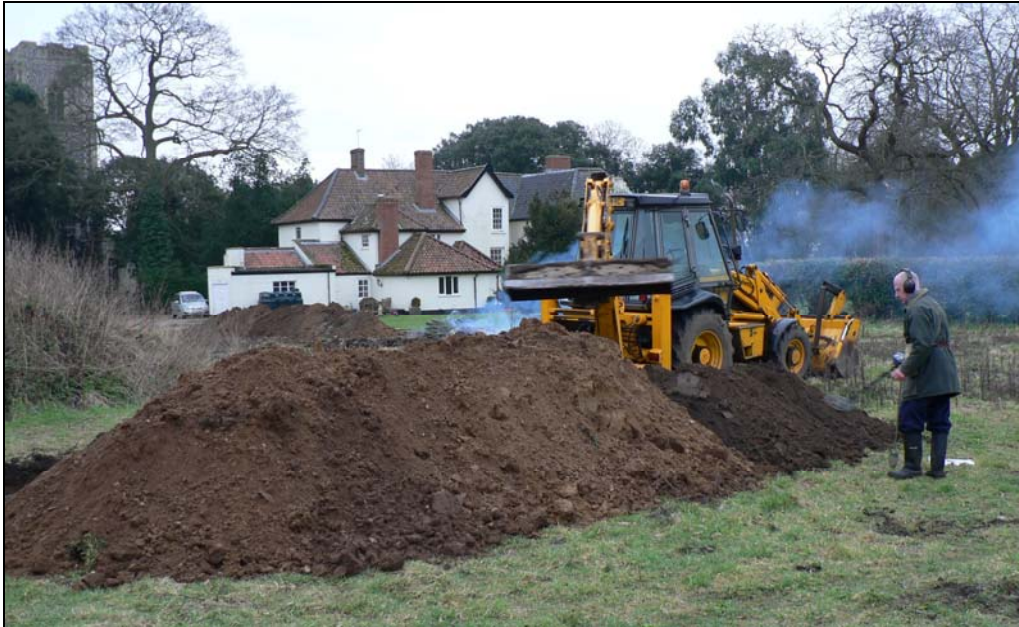
General view of from north-west
