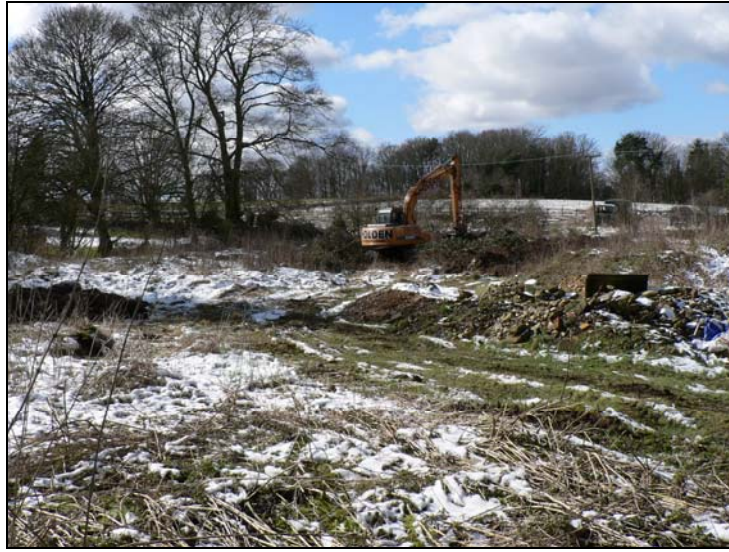
General view from north-east
