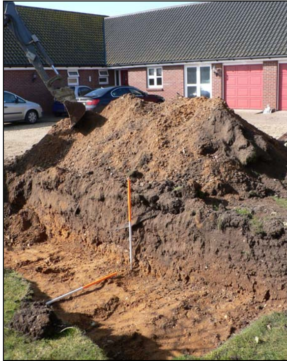
Trench from north-east
