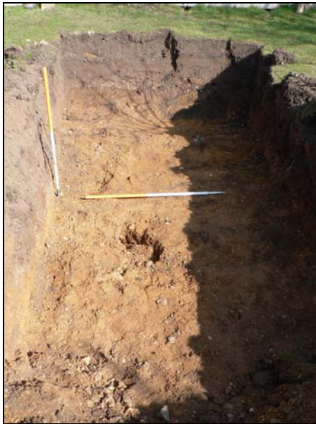
Trench from south
