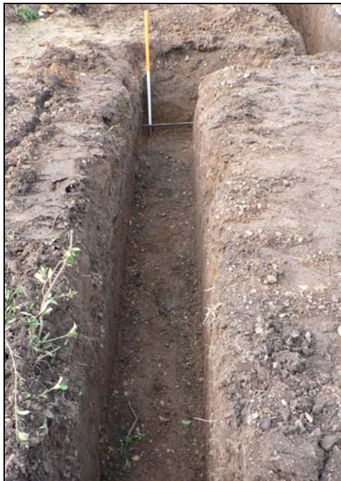
Southern foundation trench from east
