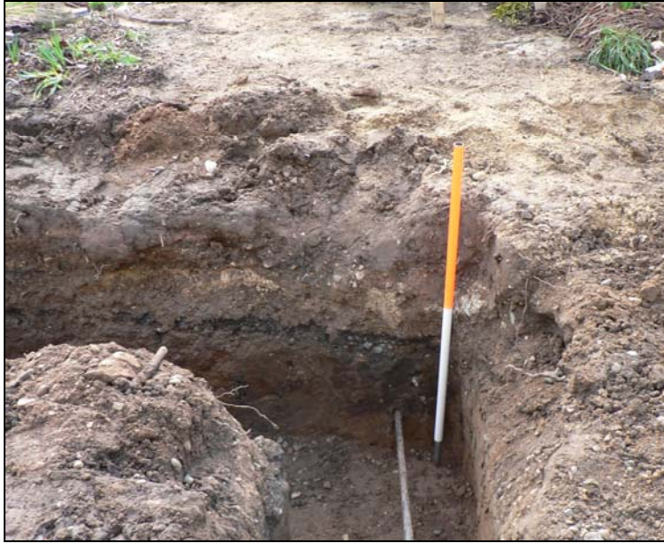
Southern foundation trench deposit profile with tarmac surface at 400mm depth
