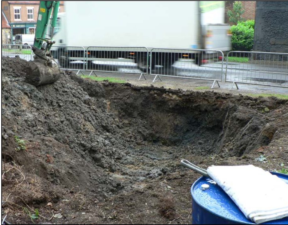
Tank removal pit from north
