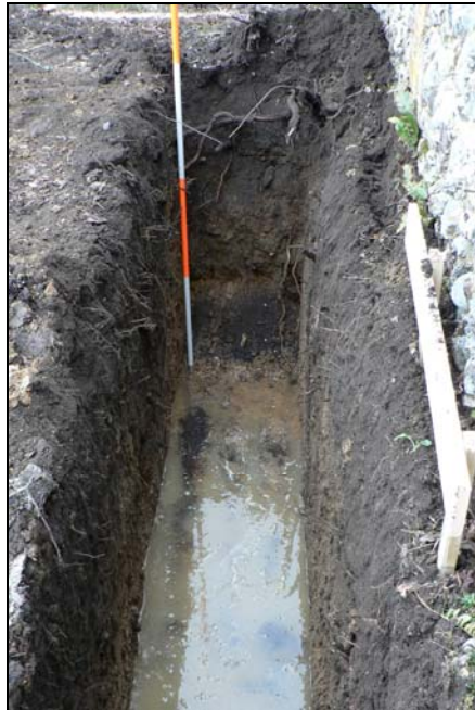
Foundation trench on east side of new build
