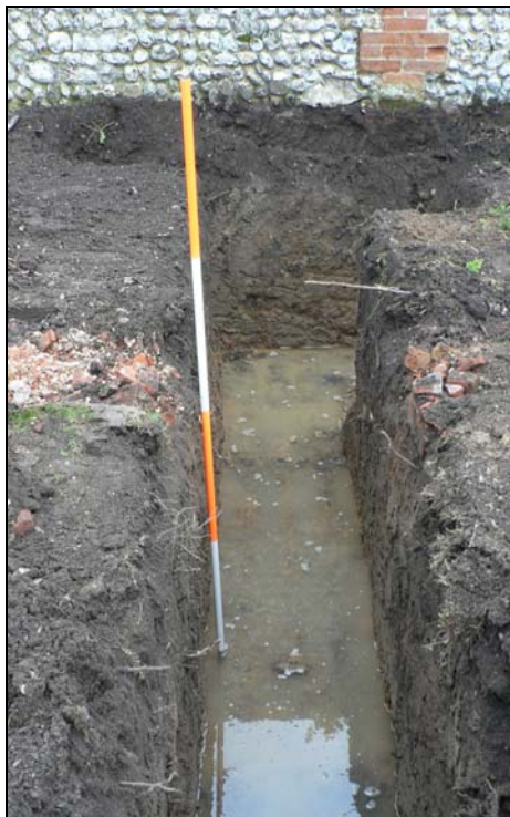
Foundation trench, north-eastern corner
