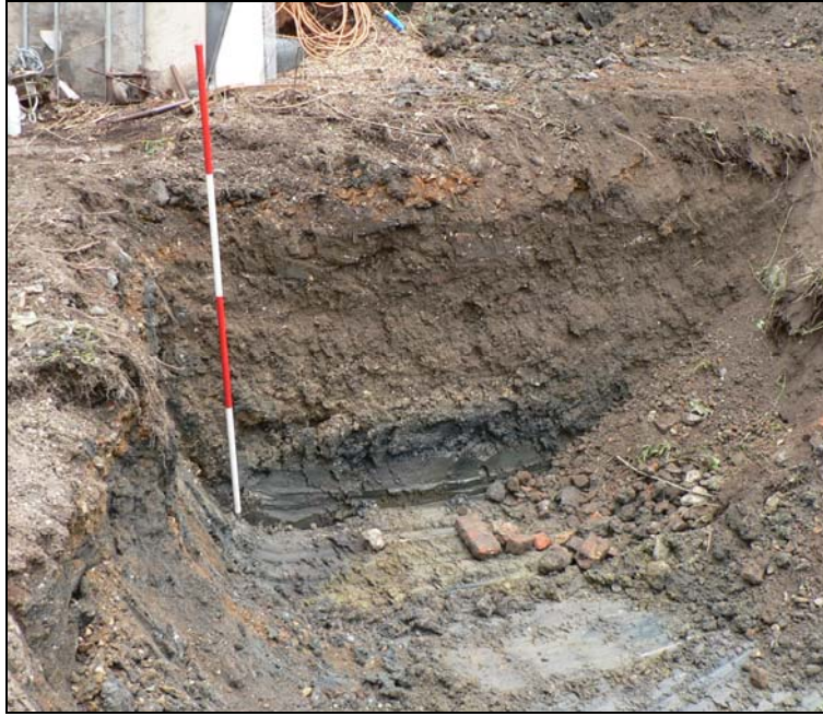
Removal of fuel tank, view from south
