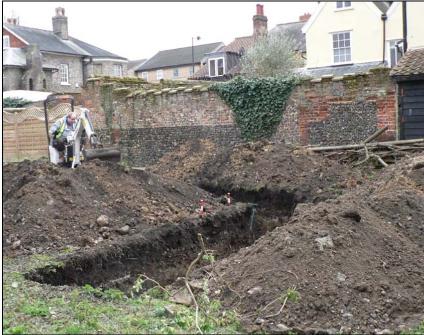
General view from north-east
