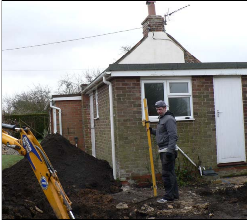
General view from north
